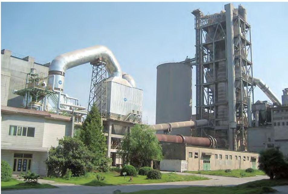
Waste heat recovery power generation system for cement plants for China
